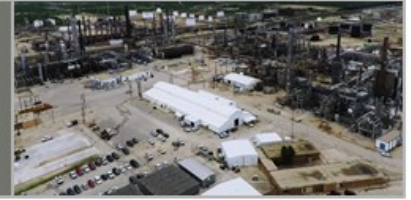
Big Spring Alon Refinery
